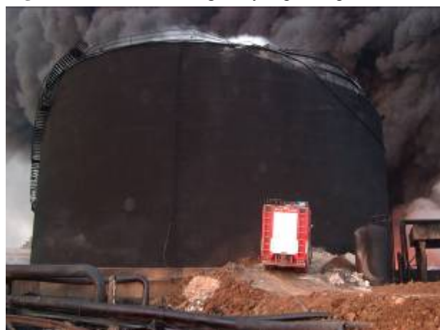
Figure 6.1 Fuel oil burning at Jiyeh power plant.
